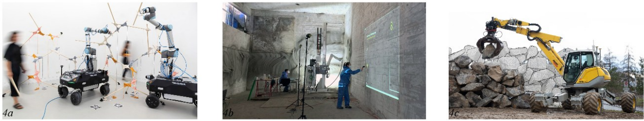
Figure 3: Pictures showing fabrication process in:
