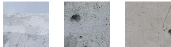
Figure 6: Example of uncracked concrete images (Tomaszkiewicz & Owerko, 2023b)
