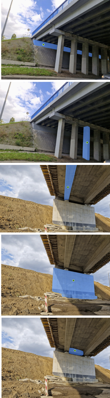
Figure 7: Results of bridge element segmentation
